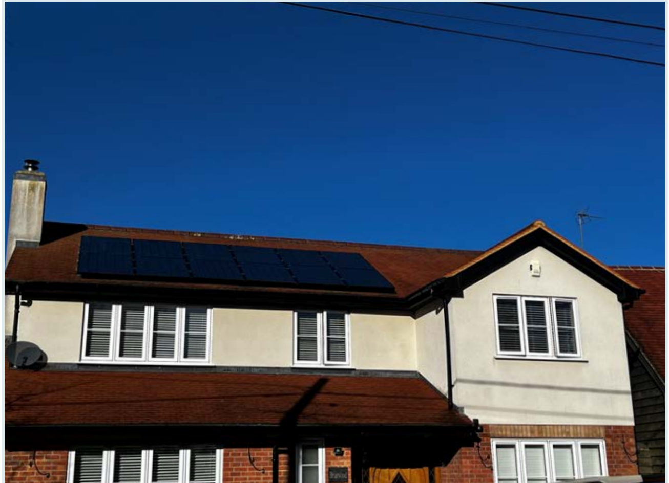
Figure 52: Local example of the use of rooftop solar panel, Amesbury Road.
