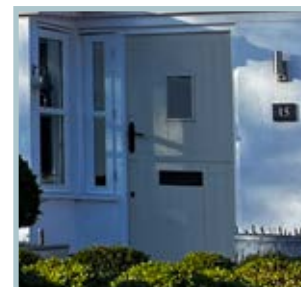
Stepped back entrance with lightly painted timber door
