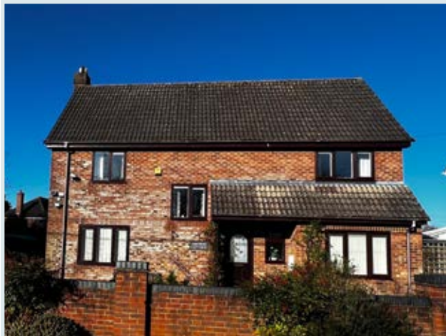
Figure 22: Front porch extension that is in-keeping with the use of material and roofline of the original property, Amesbury Road.
