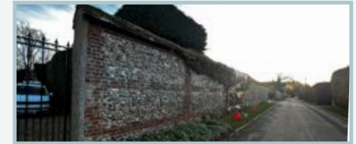
Flint stone wall with red brick detailing
