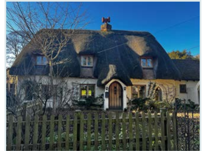
Figure 20: Positive use of matching render over brick in a side extension and dark tiled roof to create a seamless transition with the original cottage, Wiremead Lane.
