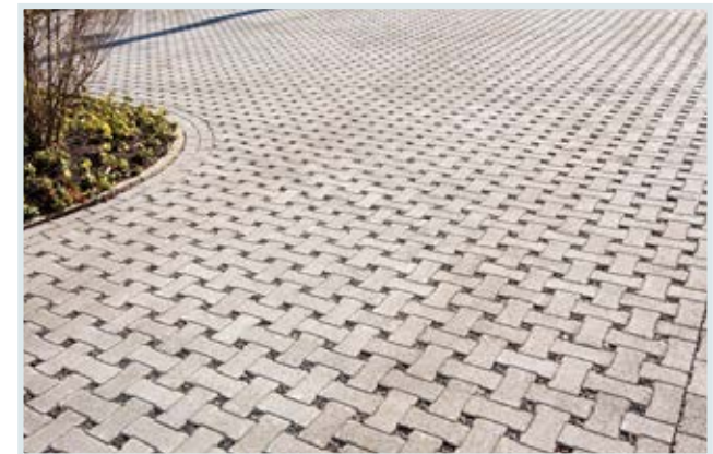
Figure 47: Example of a permeable paving that could be used for driveways.
