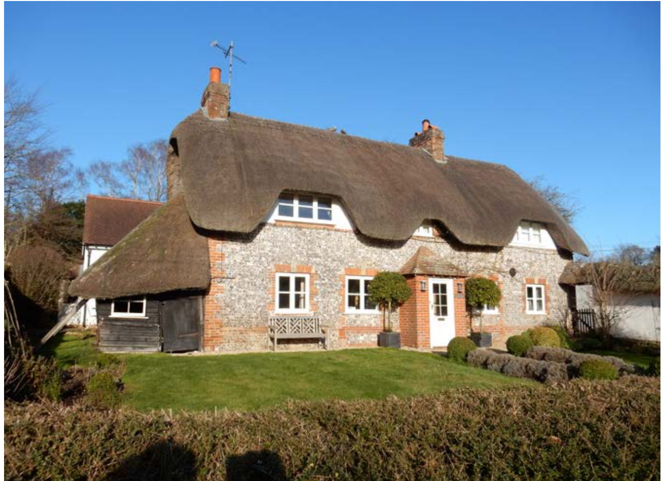
Figure 05: Local example of a traditional cob cottage with thatched roof, Amport village.
