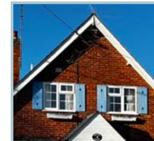
Casement windows with timber shutters
