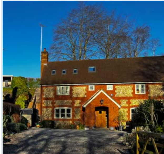
Figure 35: Sympathetically designed infill property on Sarson Lane, demonstrating the use of flint stone with decorative red brick quoins detailing which corresponds with adjacent historic properties in the conservation area.
