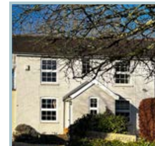
Well-positioned PVC sash windows
