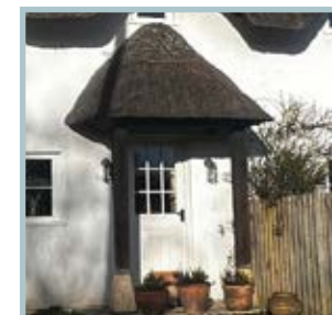
Thatched open porch with white timber door that blends in with the dominant facade
